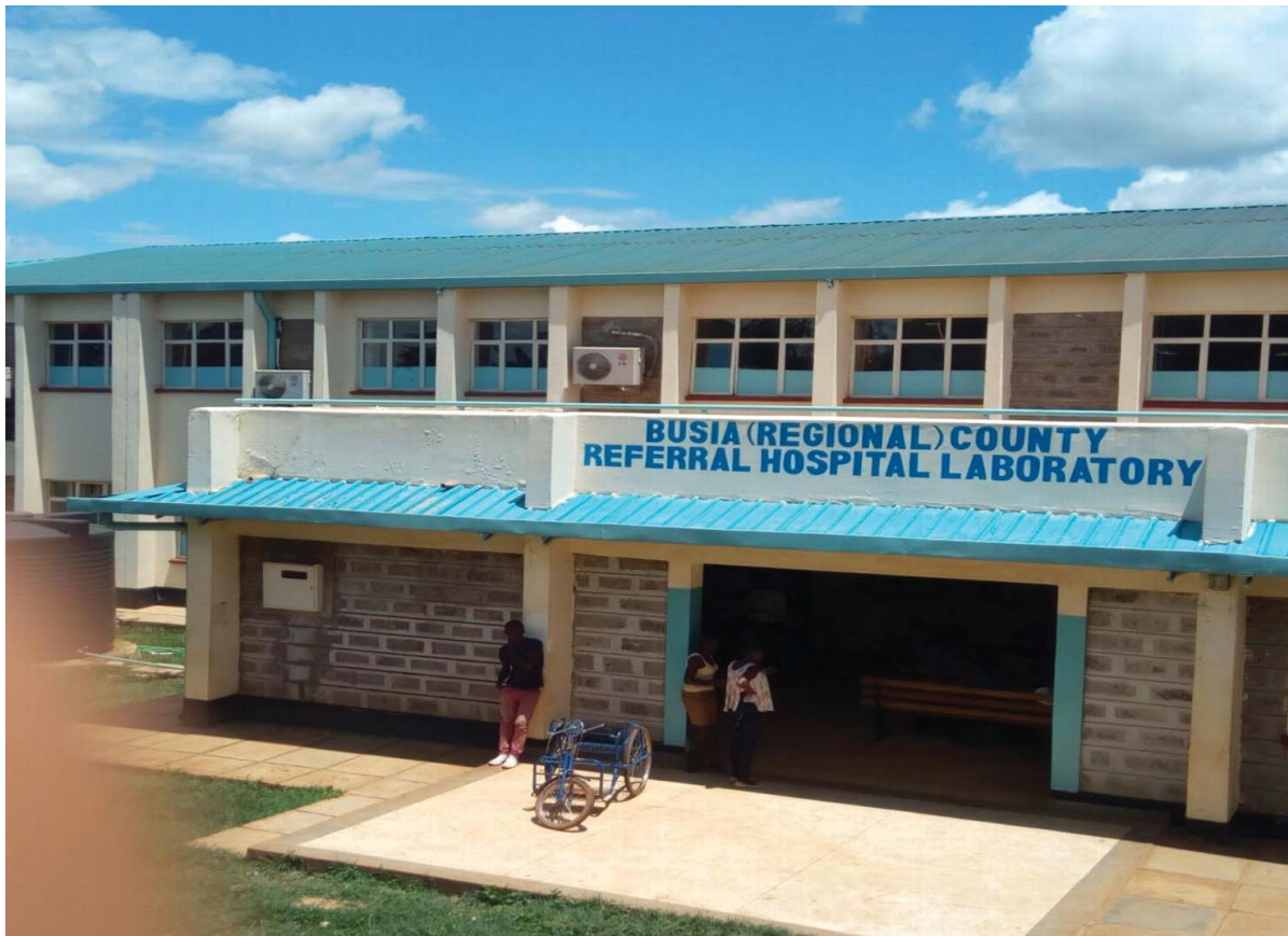
Figure 4.9 Constructed Busia Regional Public Health Laboratory
