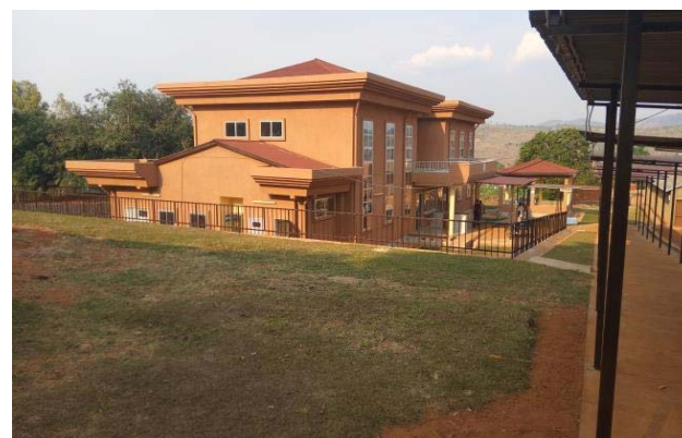
Figure 5.2 Makamba Satellite Laboratory after the Project
