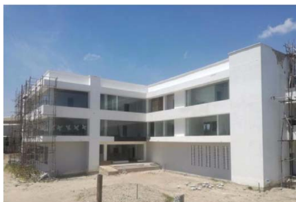
Figure 4.7 Construction of National Public Health Laboratory
